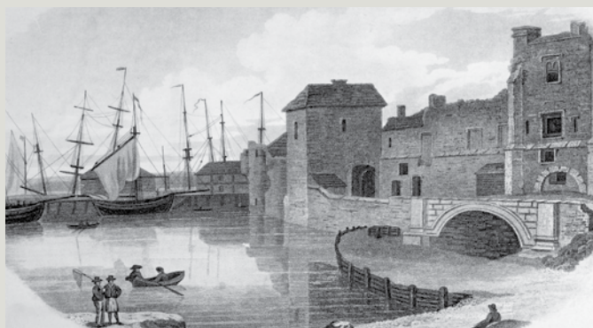
The culvert at God's House Tower 1817
